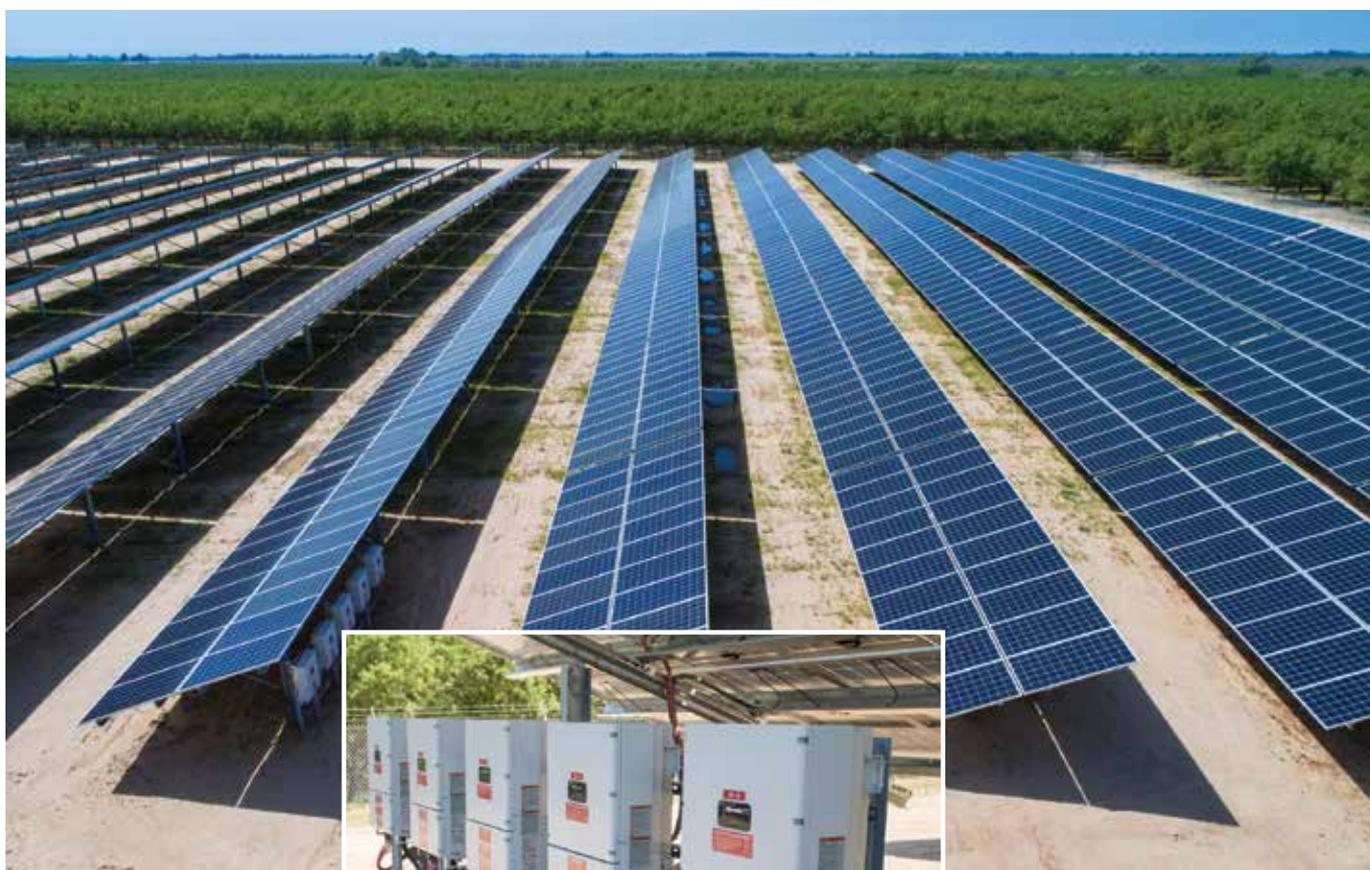
installation crew opted to build up the array pad to minimize shading from the surrounding almond trees. SunLink's PowerCare geotechnical team assessed the installation site's soils to inform foundation design and further streamline installation processes.
